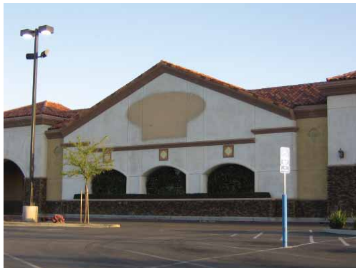
Former Ralph's at Laguna Promenade in Elk Grove
